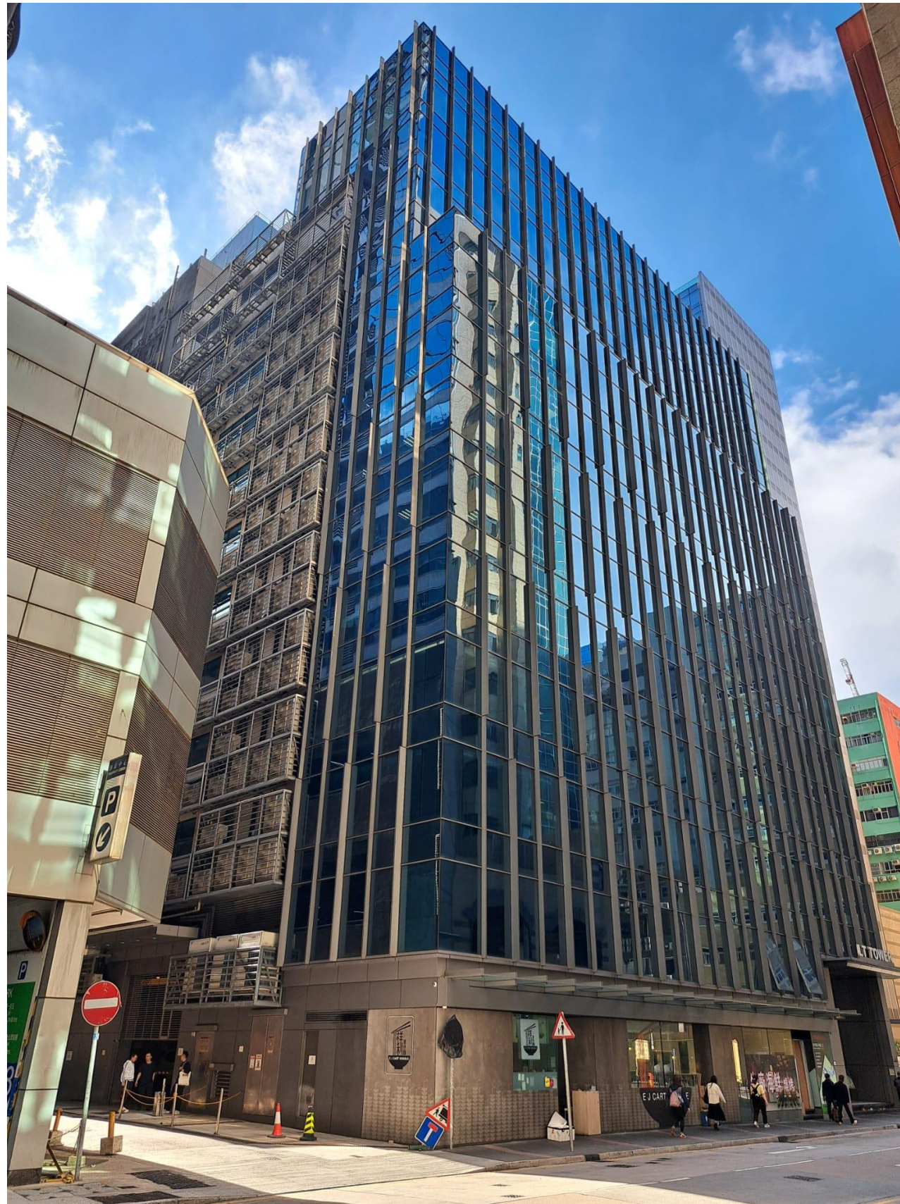
PHOTO 2 - Northern facade of the building
